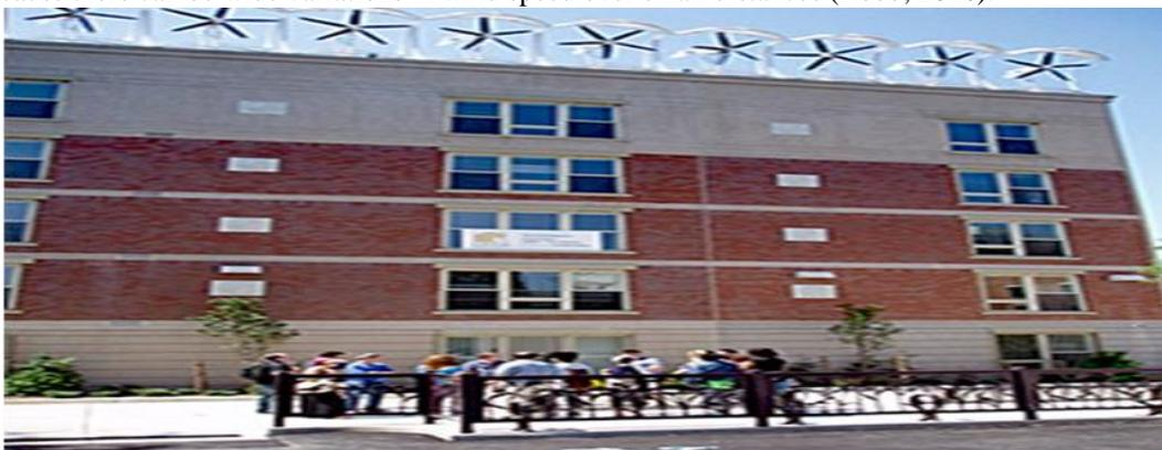
Figure 2: Wind turbine mounted all along the top of an apartment building (Robb, 2016).
